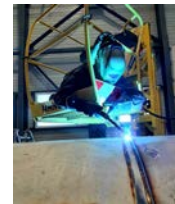
Rolled shells assembly using MAG welding process in flat position
