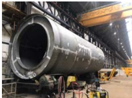
Construction of the tank in our workshop in St-Nazaire (44)
