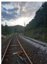
Picture of a construction site with re-use of sleepers from a high-speed line
