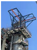
Column head structure after installation
