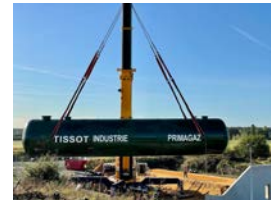
Installation using a mobile crane on site in Druye (37)
