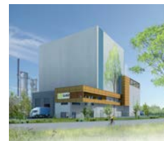
Forecast picture of the boiler.
