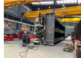
1 of the 4 elements during manufacture
