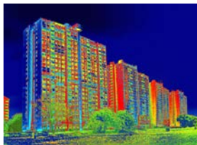
building seen with an IR thermal camera
