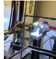
Welding of the new safety circuit line
