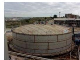
Construction of the hydrocarbon storage tank "A005"
