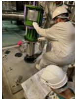
Mechanical pump installation
