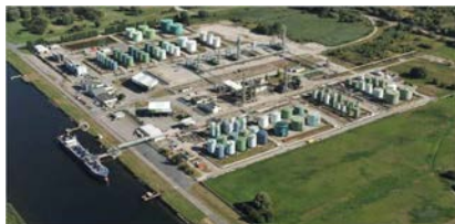
Picture of the oil depot of Oudalle
