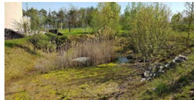
Picture 2 : Vegetated retention basin
